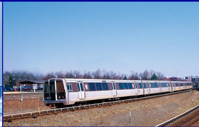
Dulles Corridor Metrorail Project
