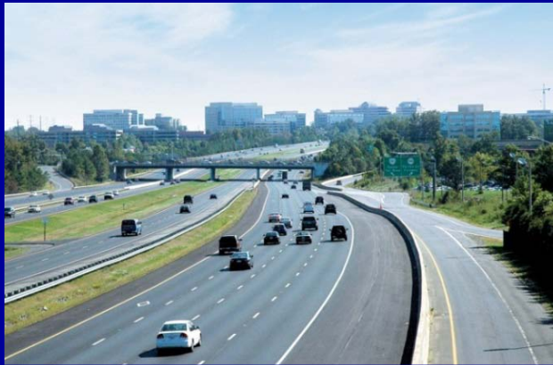
Dulles Toll Road
