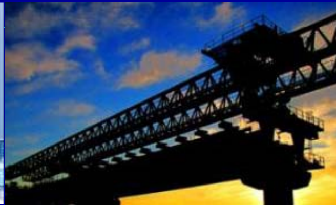
Dulles Corridor Metrorail Project
