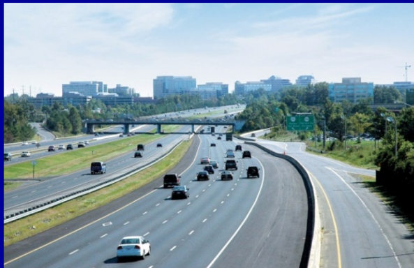
Dulles Toll Road
