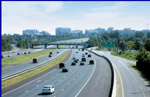
Dulles Toll Road
