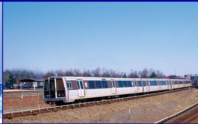
Dulles Corridor Metrorail Project
