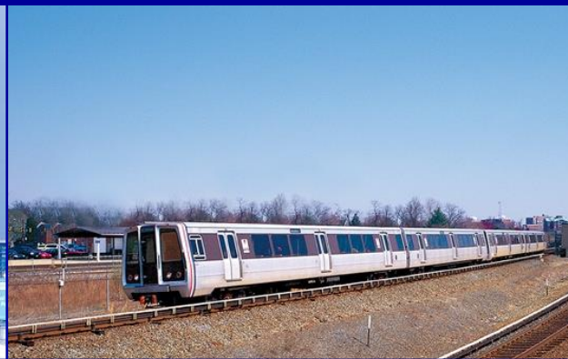
Dulles Corridor Metrorail Project
