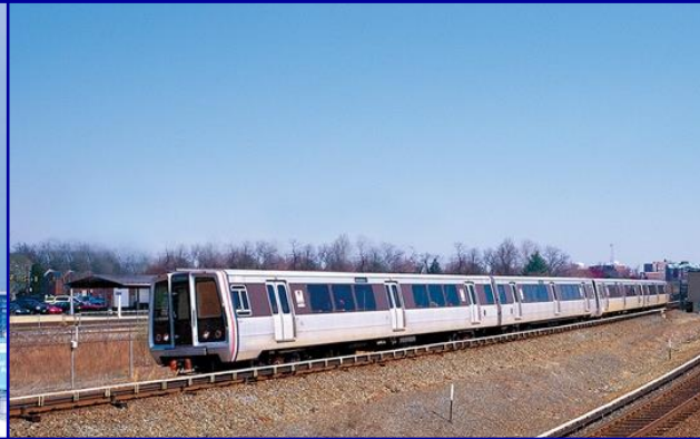
Dulles Corridor Metrorail Project
