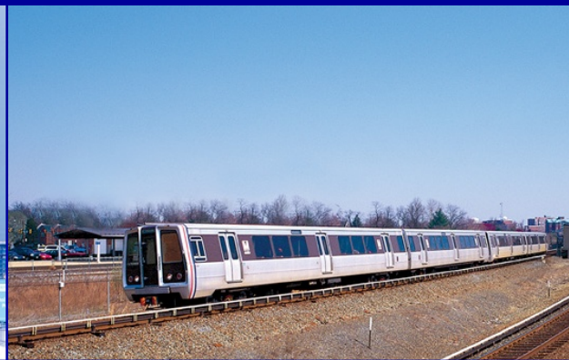
Dulles Corridor Metrorail Project
