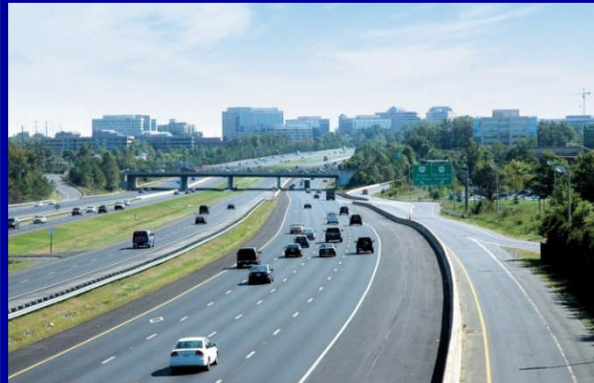
Dulles Toll Road
