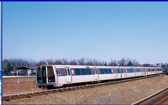
Dulles Corridor Metrorail Project
