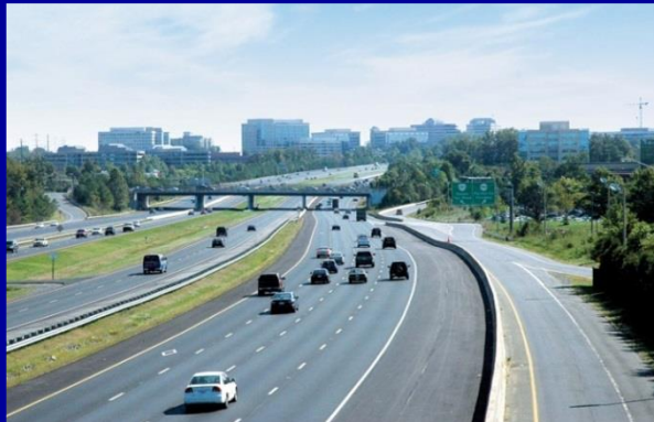
Dulles Toll Road
