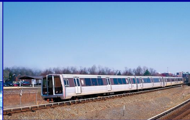
Dulles Corridor Metrorail Project
