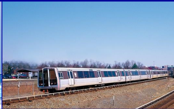
Dulles Corridor Metrorail Project
