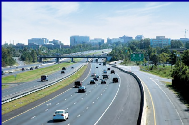
Dulles Toll Road
