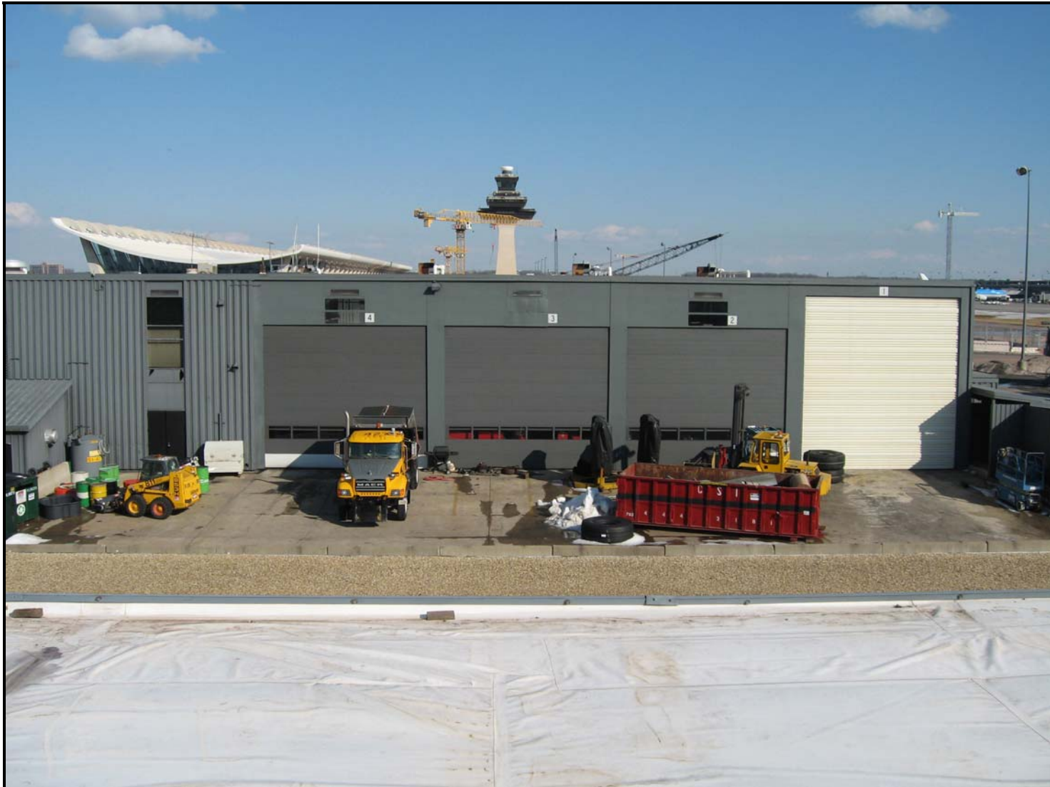
Figure 8: Shop 1 Building (Showing both sets of replacement doors)
