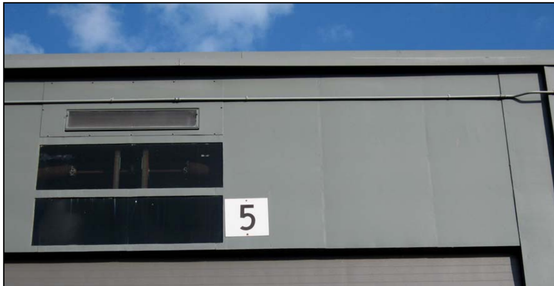
Figure 7b: Shop 1 Building (Showing details of non-original Door 5 transom)
