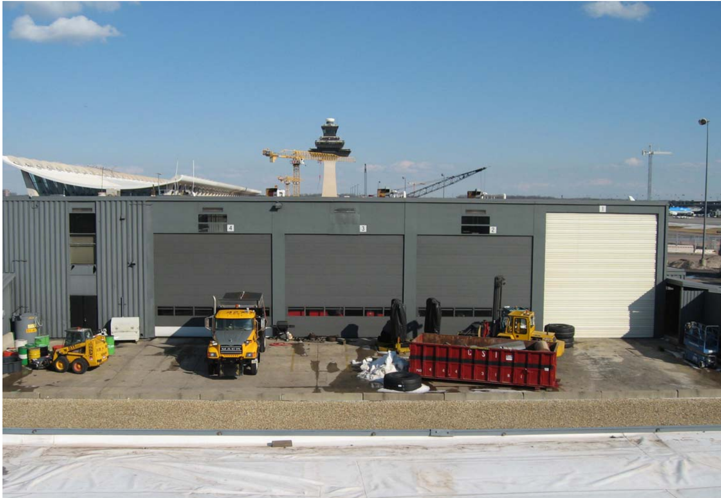
Figure 6: Shop 1 Building (Showing both sets of replacement doors)
