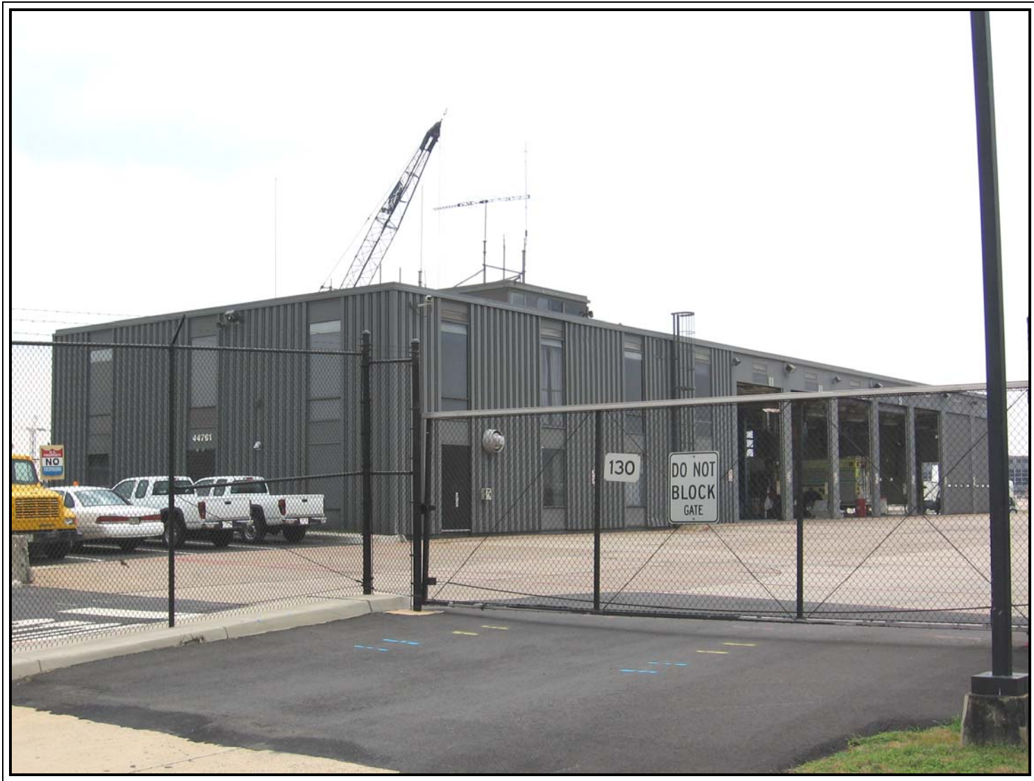
Figure 4: Existing Conditions – Shops 1 Annex
