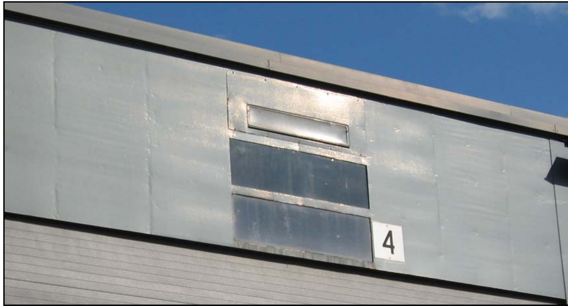
Figure 7a: Shop 1 Building (Showing details of original Door 4 transom)
