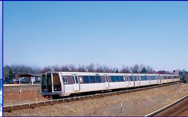
Dulles Corridor Metrorail Project
