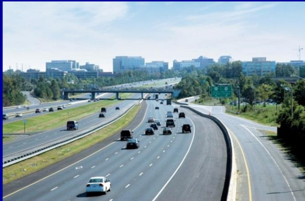
Dulles Toll Road
