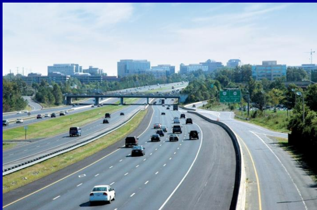
Dulles Toll Road
