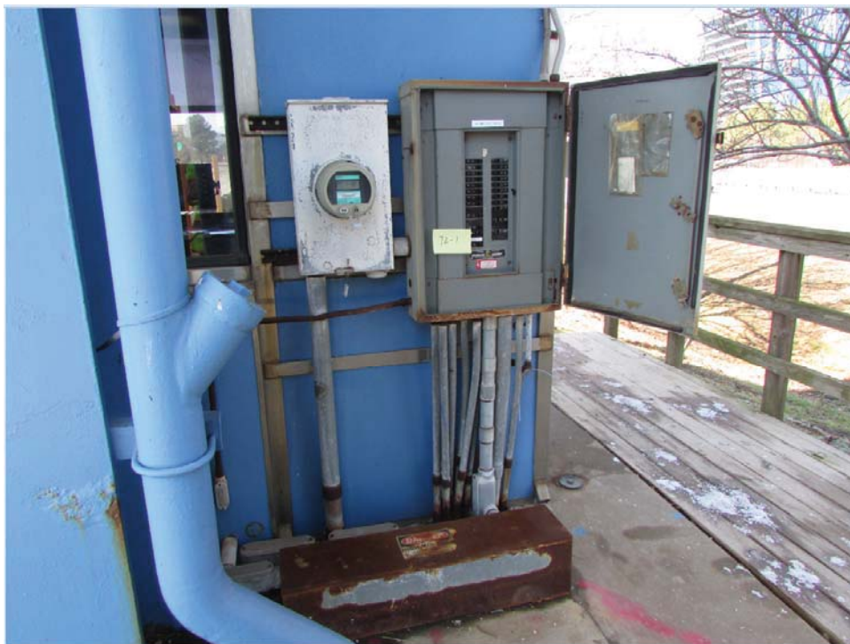
Figure 1.0 A Typical Rusty Panelboard attached to Toll booth
