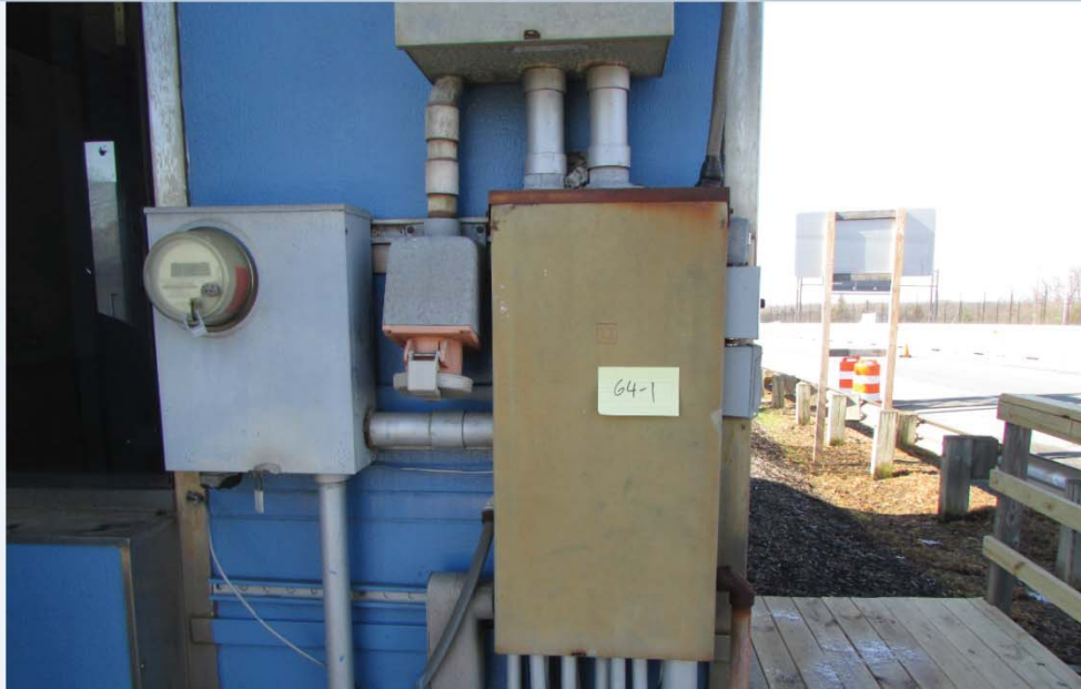
Figure 1.0 A Typical Rusty Panelboard attached to Toll booth
