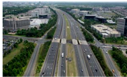
Dulles Toll Road
