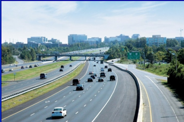
Dulles Toll Road
