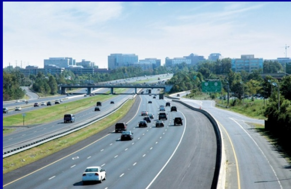
Dulles Toll Road
