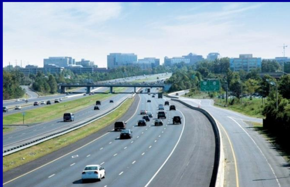
Dulles Toll Road
